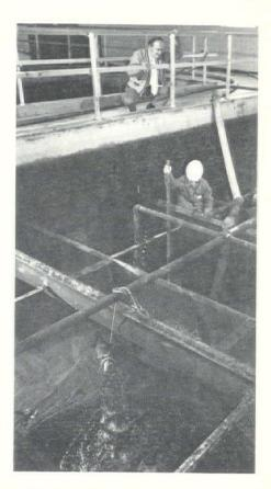
HERE COMES THE CARBON — One of eight filters at the Appomattox River Water Authority's drinking water plant in Petersburg, Virginia, is filled with a slurry of granular activated carbon supplied by Calgon Corporation, Pittsburgh. Watching the carbon fill — and anticipating drinking water free of taste and odor — is the Authority's General Manager, Robert E. Sayre.
