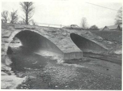
This installation is located along Route 328 near Elmira Heights in Chemung County, N.Y. The old bridge was removed and a new Lane structural plate bridge installed and backfilled within a week.
