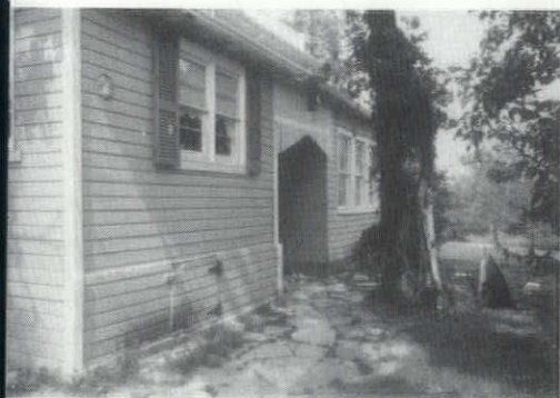
Before: Stone foundations covered, and recessed rear entrance changed character of house. After: Restructured rear of house true to Georgian style.
