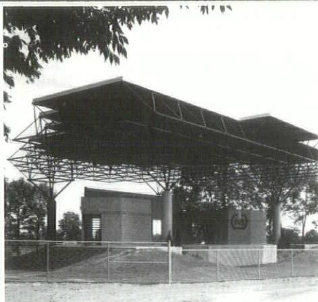
The first completed installation of Unistrut Space-Frame System II was the sound stage roof for Molson Park, Barrie, Ontario.
