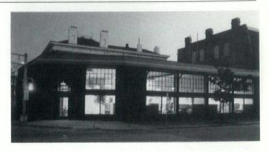
was extended to cover the entrance. The roof is clad with slate shingles laid in polychromatic pattern, common in the historic district. Applied, painted wood mouldings and the colored slate shingles were used as exterior color accents and were carried through to the building's interior color scheme.
