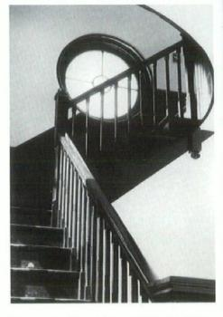
that space did not have sufficient height or width to accommodate the stair. The solution was to build half the stair within the original building, cut through the original exterior wall into the existing addition and complete the stair run within the addition.
