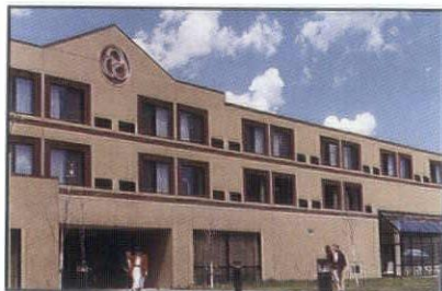
Load bearing panels
