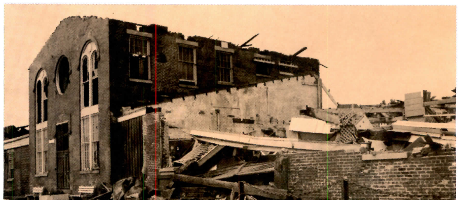
The antebellum Southside Railway Depot lost windows, portions of roof and entire east wing.
