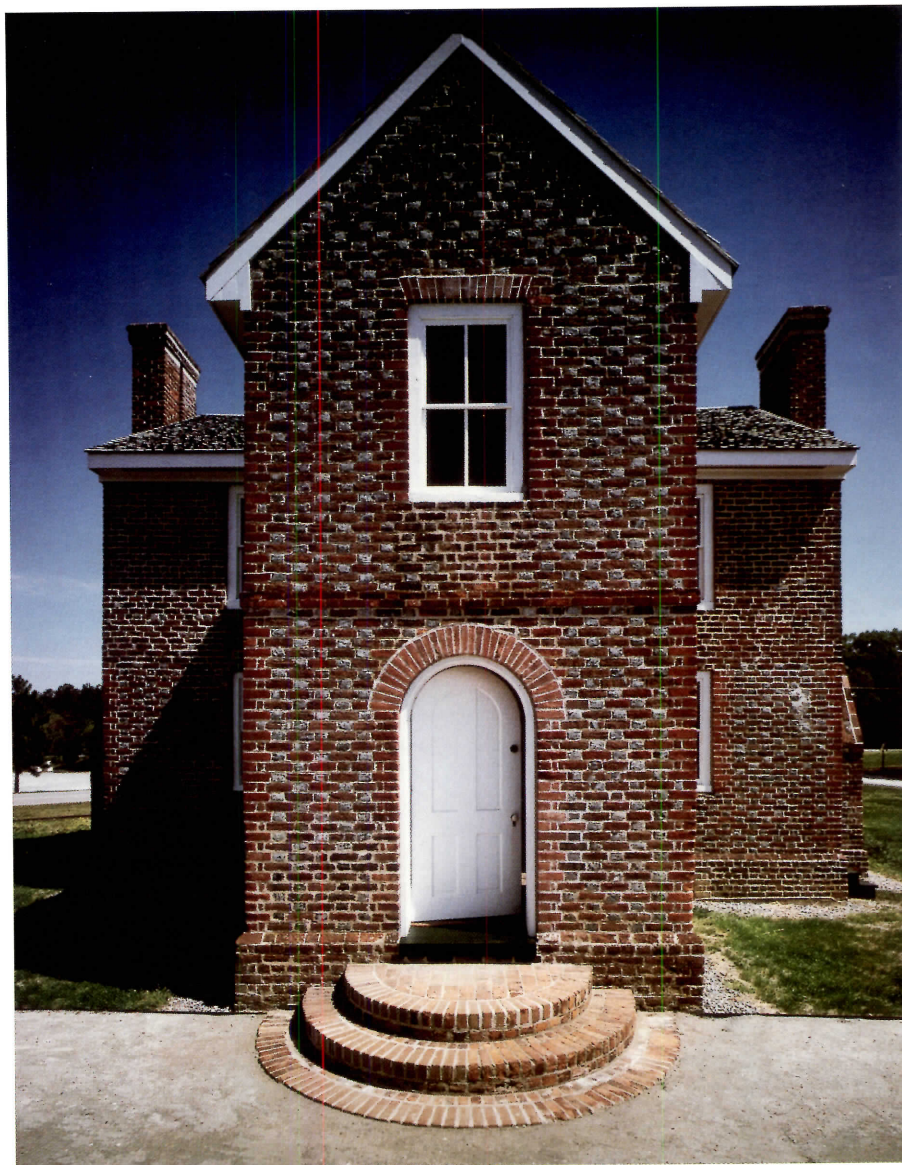
Restoration included replication of window sashes, replacing oak shingles, and duplicating original paint colors (above). Before the work began (left).
