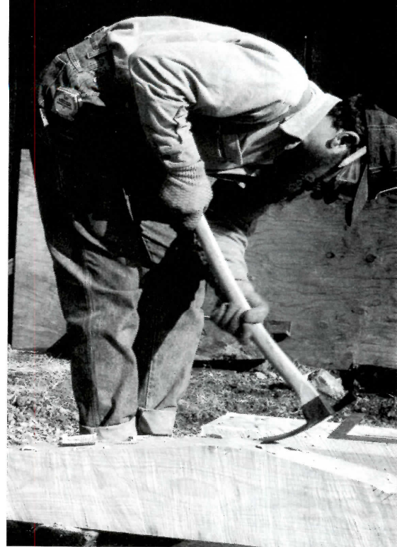
Restoration craftsman Doug Rideout shapes a lintel for one of the arched windows.
