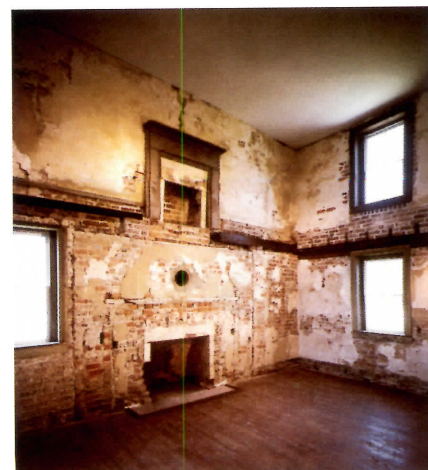
Missing second floor reveals building frame.
