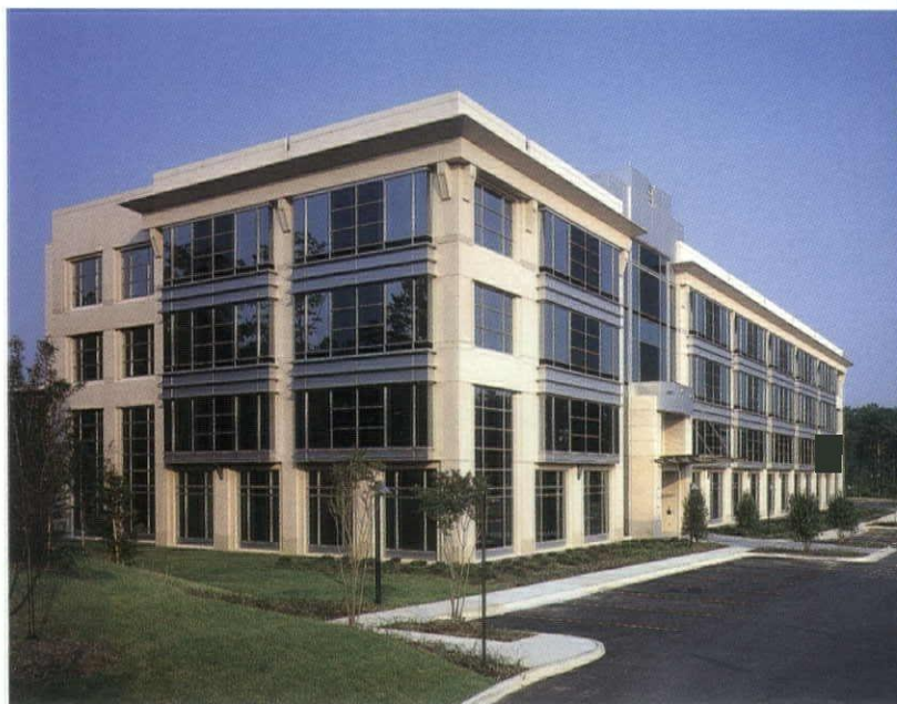
From the parking lot, the addition appears as a single volume with a skin of precast concrete and projecting glass bays (above). The dramatic stair tower and curved facade are seen when entering the site by car (facing page).
