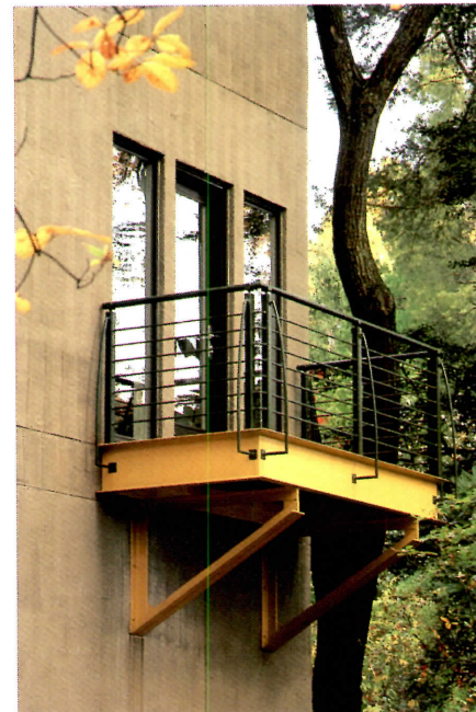
Walls are stucco over a wood frame; balcony supports and handrails are steel.
