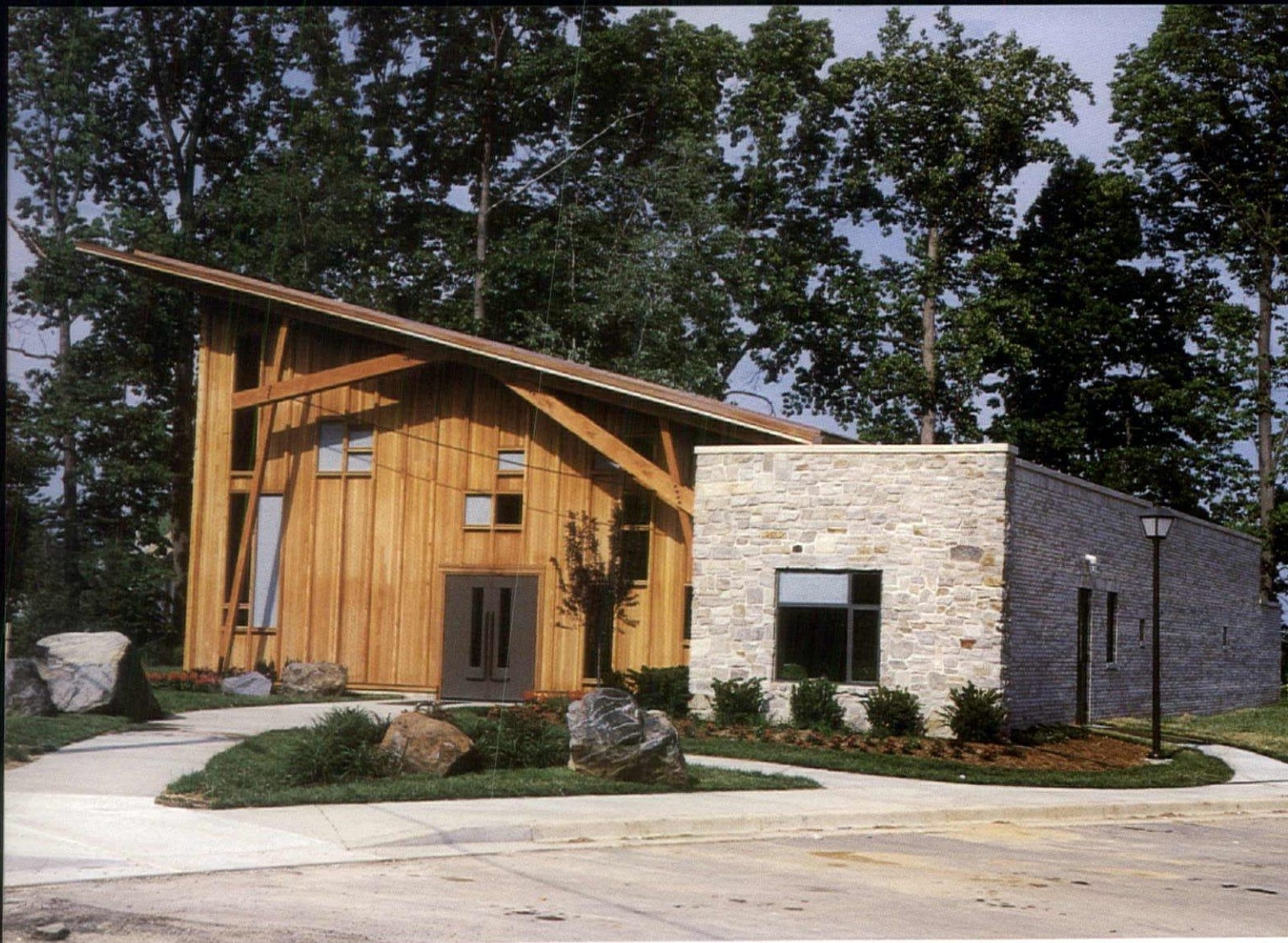
The chapel was conceived as two distinct volumes: a soaring, light-filled cedar tent and a lower, darker masonry bar (above). Heavy timber columns are set at an angle on concrete plinths whose tops are sloped to meet the angle of the wood (below).
