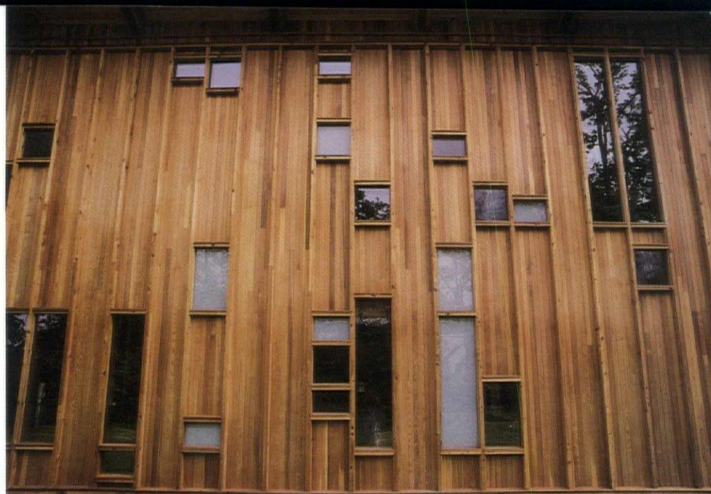
Using cedar as a building material enabled Kerns to explore the play of light inside the chapel with nonloadbearing perimeter walls that are perforated by windows (above).
