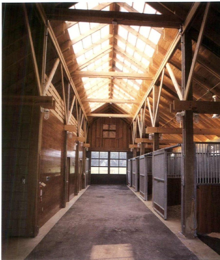
The continuous skylight, made of heavy gauge corrugated fiberglass (above), makes artificial lighting unnecessary during the day. The barn's exterior is pleasantly subdued on the horizon (left).
