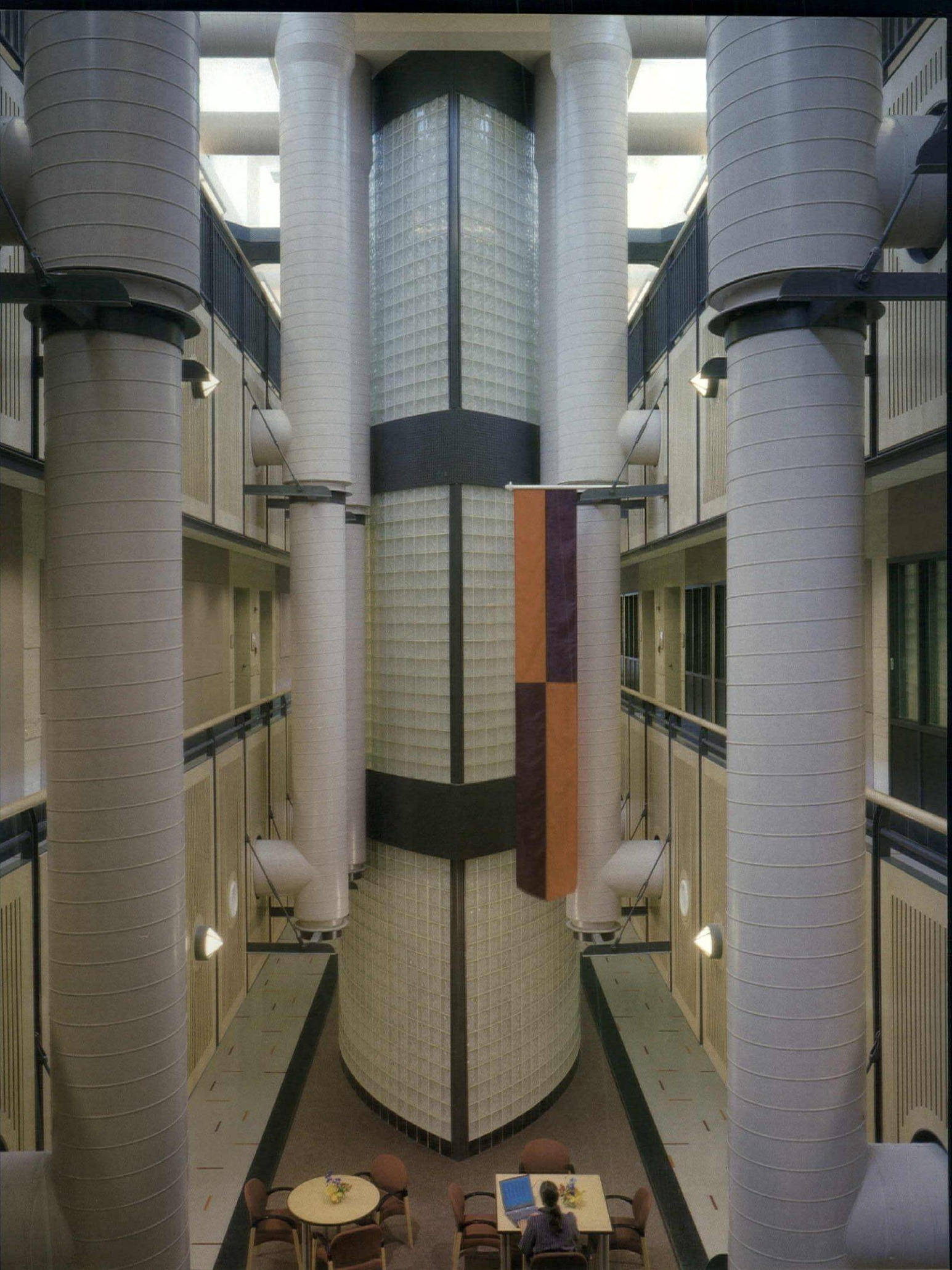
Two glass-block towers inside the building's atrium provide space for the computer network hardware and wiring.
