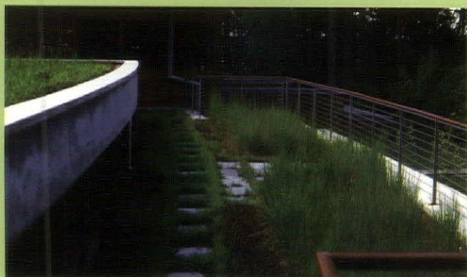
Roof garden (left) absorbs runoff and produces oxygen. Woodland walk leads to a quiet place of the suburban site (right).
