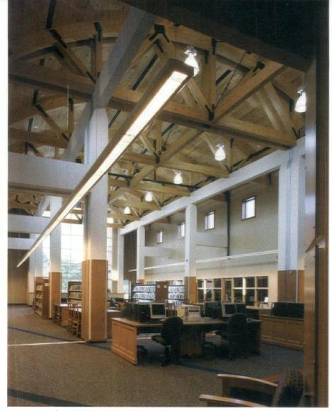
Second-floor spaces reside beneath a towering vaulted ceiling supported by stout wood-and-steel bowstring trusses.
