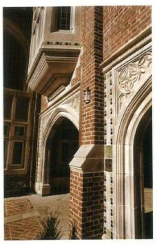
Rich limestone detailing was achieved through modern stone-cutting technology that incorporates the architect's CAD drawings.
