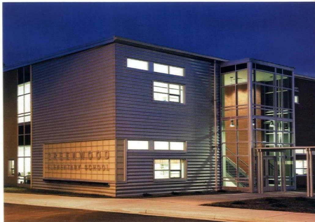
The open stairwells that lend the school distinction – and fill the hallways with daylight during school hours – are made possible by recent changes in the building code.
