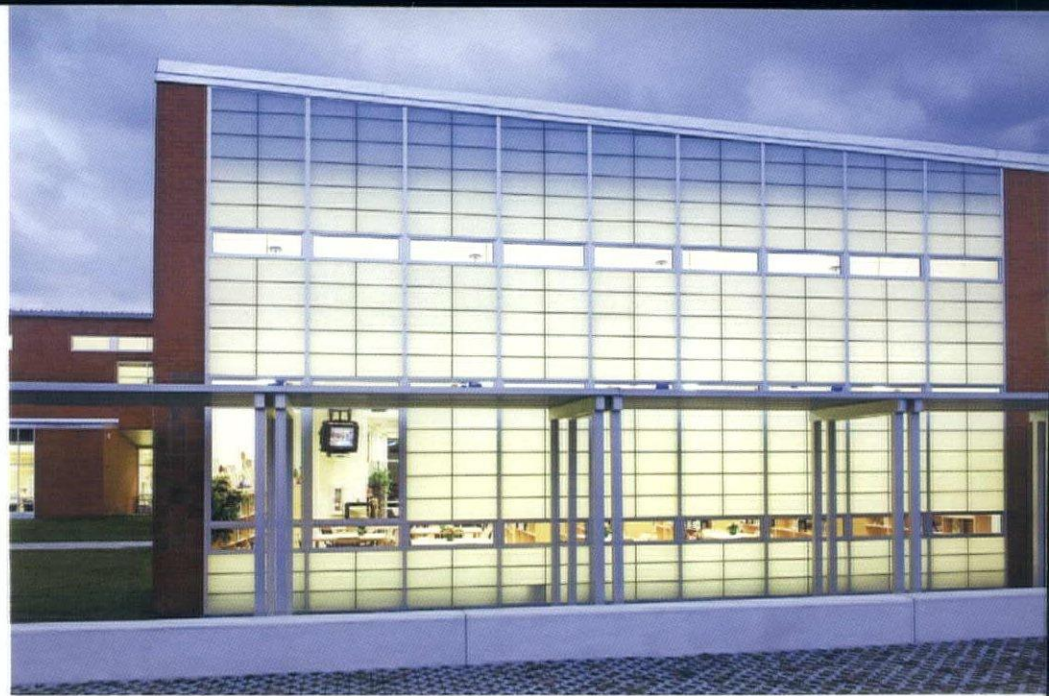
Translucent glass provides diffuse daylight during school hours and glows at night (right).
