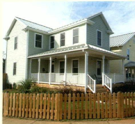
Swenson's fellowship included the construction of new affordable houses in Charlottesville.
