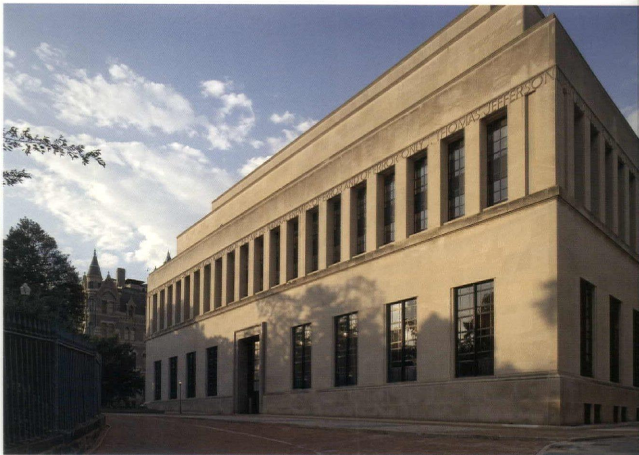
The south entry fronts Darden Plaza and faces toward the Executive Mansion. The top stories, which step back from the original façade, were added in 1970 in accordance with expansion plans conceived in the late 1930s.
