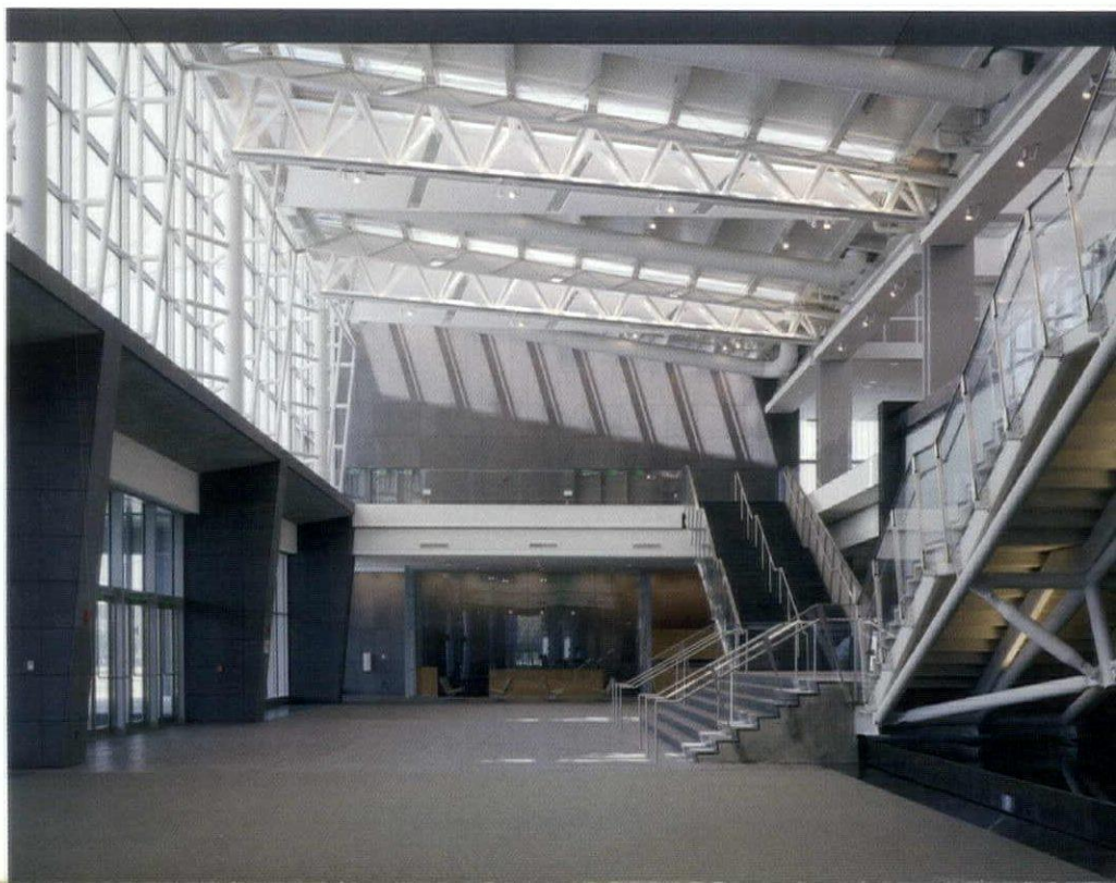
The center's lobby is a structural tour de force, with trusses supporting the roof, glass wall, and monumental stairs (below). The effect is more subtle in places such as a stairwell (above).
