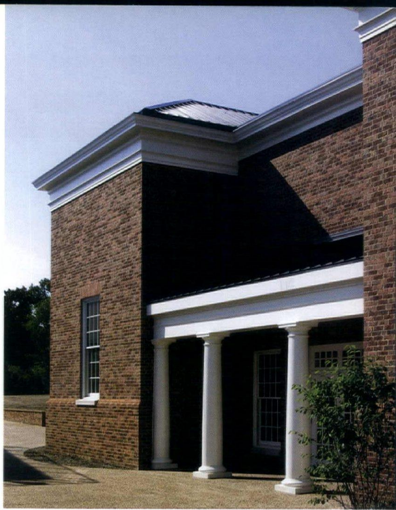
To avoid overwhelming the campus, the athletic center's mass is modulated by varied roof forms, deep entablatures, and shallow colonnades.
