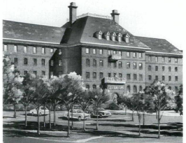
Architect: BeeryRio, Springfield Project: Long and Foster
