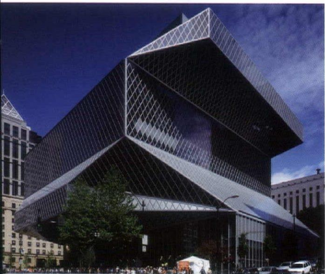
The Seattle Central Library combines structural steel and glass in eight horizontal layers. The striking landmark was designed by Rem Koolhaas' architecture firm, Office for Metropolitan Architecture.
