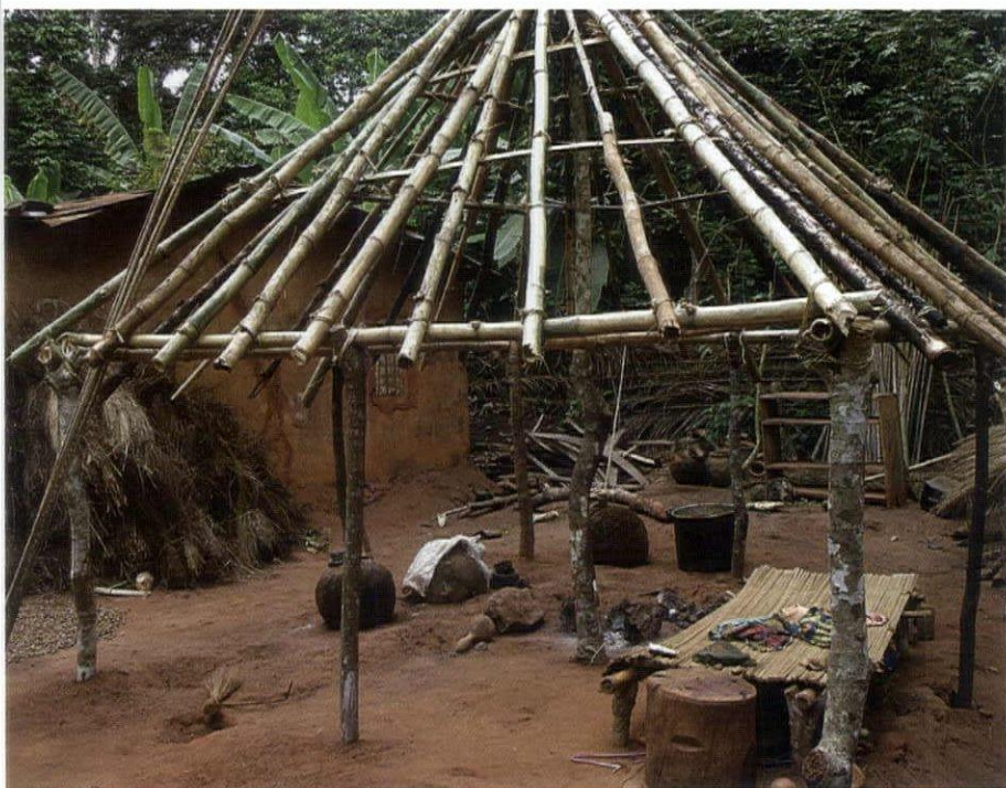
A dwelling under construction in an Umuoka village, Enugu State, Nigeria, showing the basic frame that would inform the Frontier Culture Museum how to construct an authentic West African village.
