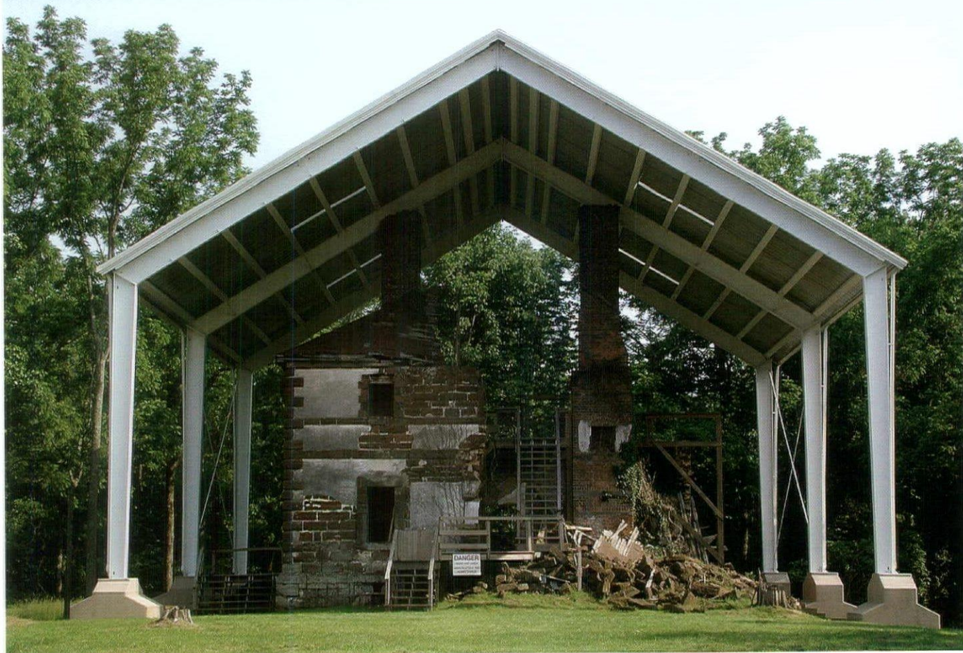
Menokin's temporary shelter has been an imperfect solution to the issue of protection. While its basic coverage has provided researchers coverage from the sun, precipitation continues to affect the structure.
