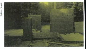
The Pope-Leighey house under construction in 1940 (above). The three masonry piers provided support for the roof and allowed the open plan typical of early Usonians.
