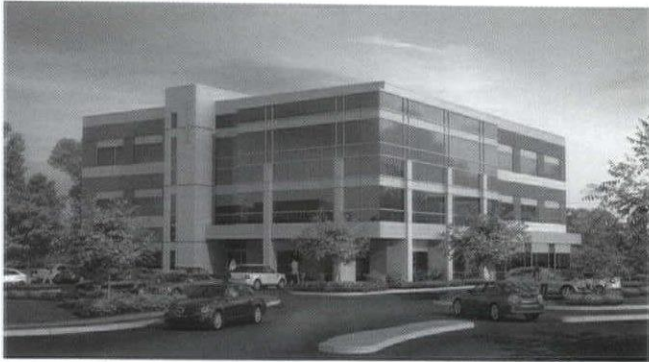
Architect: INNOVATE Architecture & Interiors, Portsmouth Project: 1168 First Colonial Medical Office Building, Virginia Beach
