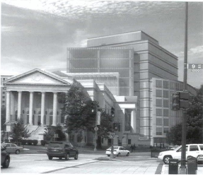
Architect: SmithGroup, Washington, DC Project: 901 K Street, Washington, DC
