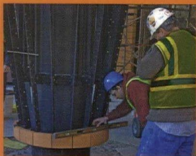
One of the Museum's most distinctive features is the terra cotta cladding, which had to fit precisely.
