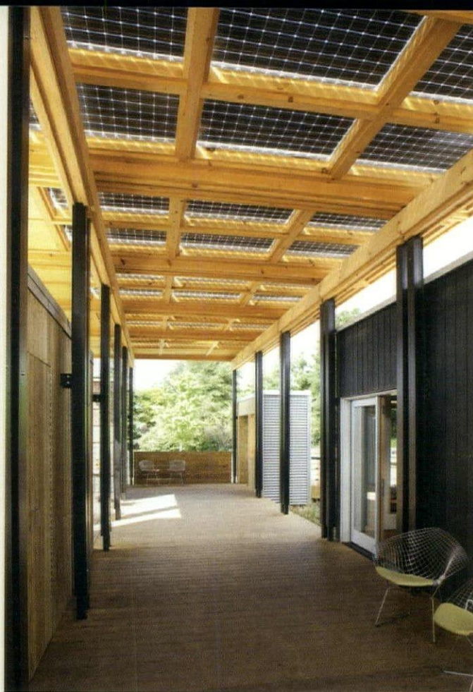
PV-panel shaded breezeway of the Appalachian State U. Solar Homestead.
