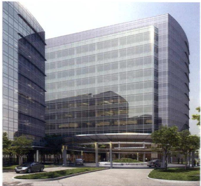
Architect: ODELL Project: Research Forest Lakeside, Buildings 4 and 5, Woodlands, Tex.
