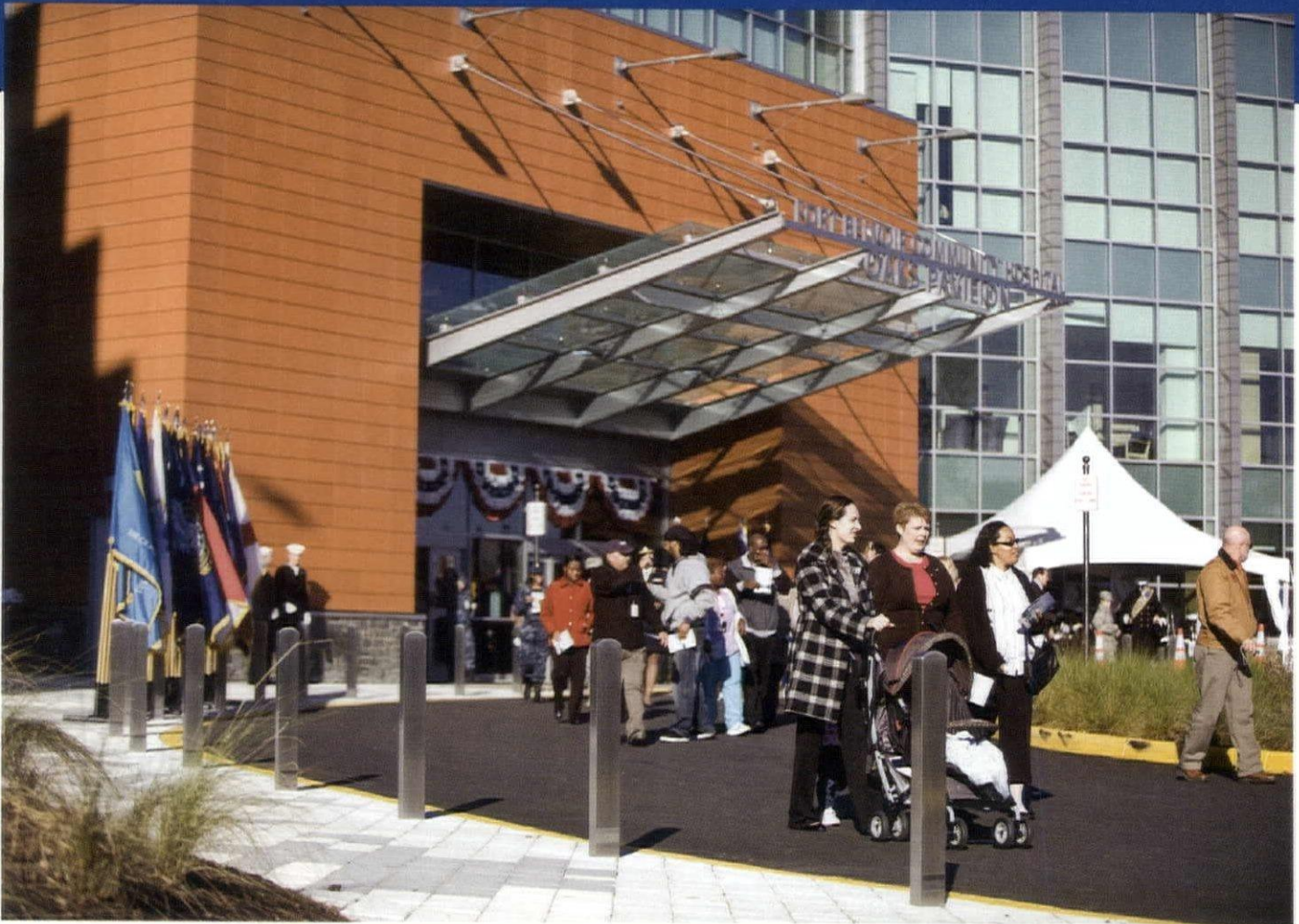
Among the buildings Clark-Nexsen has reviewed for its healing qualities is the Fort Belvoir Joint Hospital Center (see pages 16-21), here seen on its dedication October 28.
