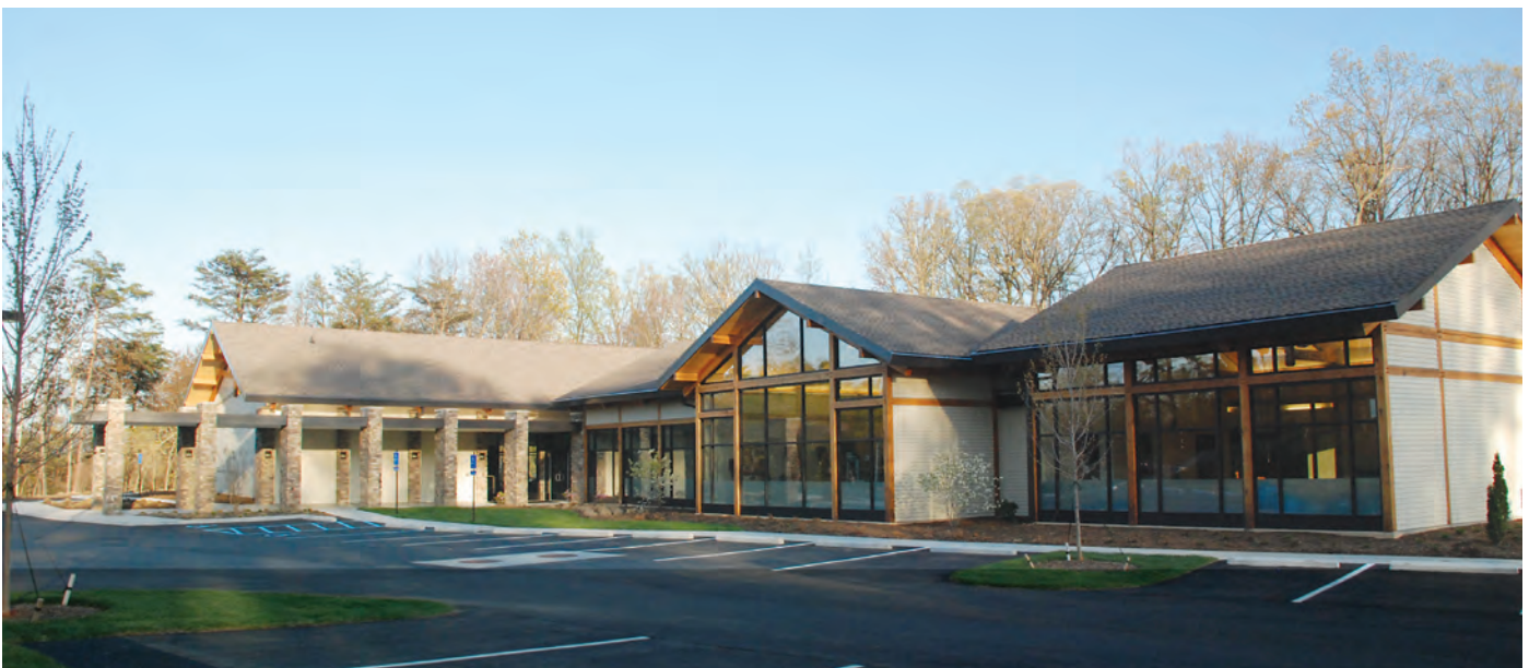
Heavy timber beams and faux-stone column covers evoke the Appalachian setting of the Warm Hearth Village. Teams of draft horses helped harvest trees from the site.
