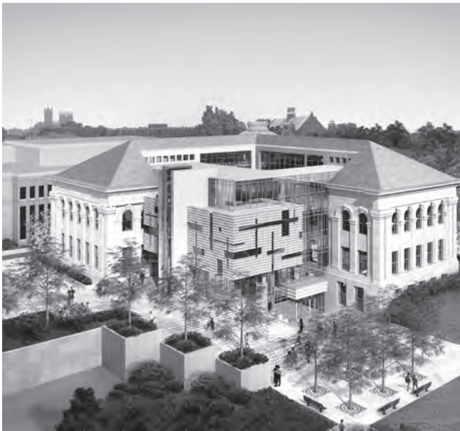
Architect: Bowie Gridley Architects, Washington Project: American University—McKinley Hall, Washington
