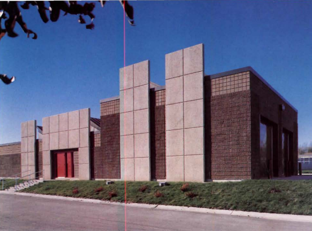
The complete building showing the split ribbed and scored concrete masonry units used for the exterior.
