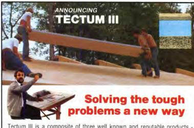
Tectum III is a composite of three well known and reputable products -Tectum, Styrofoam\* brand insulation (which is water resistant), and waferboard. The synergistic effect is the new product has much more structural strength than any of the individual products, and retains the key physical properties of each to make a superior overall building product - and Tectum III is easy to install. Three thicknesses available.
