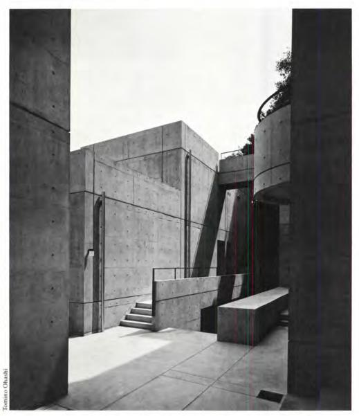
A master craftsman of reinforced concrete, Ando creates a procession of curved walls, asymmetrical stairs, each with a different number of steps, leading to terrace entries on roof of apartment below that allow visual contact between neighbors.
