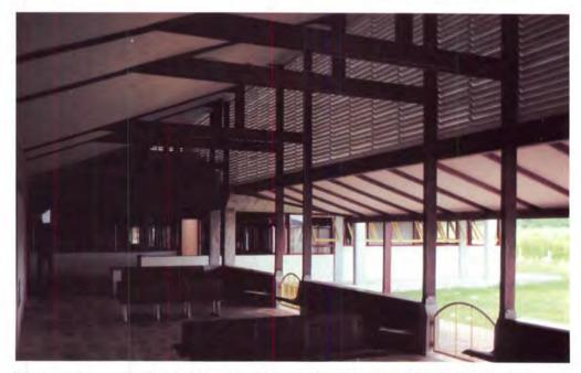
Deep overhangs, bands of wind scoop-like louvers largely obviate airconditioning.
