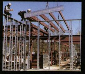
The need to build fast and economically, combined with a poor soil-bearing site and a 4-story design that required non-combustible wall, floor and roof-truss systems . . . all added up to one best solution: lightweight steel framing by Inryco.
