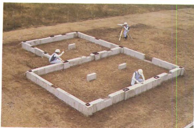
Above, conventional poured-in-place concrete footings support prefabricated volumes, which are transported to the site on trucks. Right, local subcontractors, affiliated with Misawa, hoist volumes from truck using a separate crane. Most houses are comprised of seven to ten volumes. The size of each volume is limited by road transportation restrictions.
