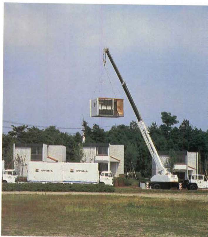
Above, conventional poured-in-place concrete footings support prefabricated volumes, which are transported to the site on trucks. Right, local subcontractors, affiliated with Misawa, hoist volumes from truck using a separate crane. Most houses are comprised of seven to ten volumes. The size of each volume is limited by road transportation restrictions.
