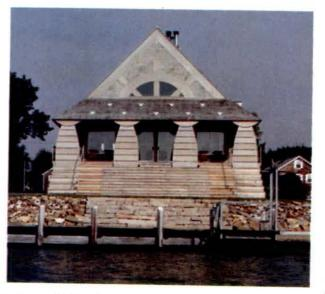
size, this is essentially a one-story house. The ground level is devoted to a cozy foyer, garages, and utility rooms. The house is constructed on piles to which the upper structure is bolted, allowing the bottom enclosure and the south steps to break away in the event of a flood.
