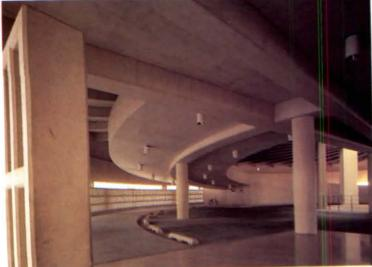
T-shaped concrete slabs with precast inserts were used to cover the steel framed structure.
