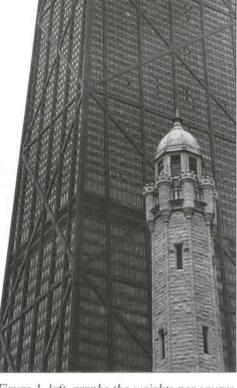
Figure 1, left, graphs the weights per square foot of steel needed for floors, columns, and wind versus number of floors in a building. Chicago's Hancock tower, above, was designed to keep these steel requirements to a reasonable level. Figure 2, below, compares actual stress due to shear lag versus true cantilever stress.
