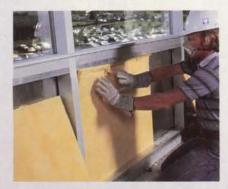
mance in exterior walls. Made from bonded glass fibers with or without selected facings, it delivers superior R-values or K-values when compared to rockwool insulations of much higher density and weight.
