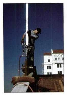
Workers core a masonry wall prior to placing and grouting rebar for seismic compliance.
