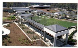
Galvalume sheet offered the Center's architects a way to precisely and cost-efficiently match the color of the arcade roof to the building's charcoal gray trim, enhancing the visual unity of the Center's landscaped approach, arcades and main building.
