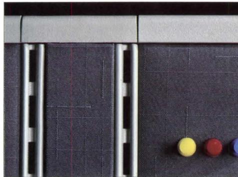
door frames, glazing, and other components are prefinished aluminum extrusions. The system is available in three profiles: Projected, with a rectangular form extending out from the wall surface; Flat; and Radius Profile, which uses extrusions with a rounded exterior form. Optional panel connectors are designed to support storage components and work surfaces.
