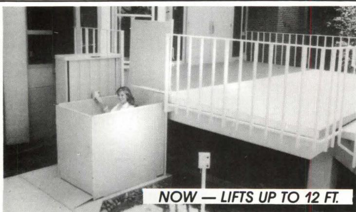
Whether you're modifying an existing building or designing a new one, accessibility to the handicapped is important. And PORCH-LIFT provides the simple, economical solution . . . indoors or outdoors. This safe vertical wheelchair lift platform anchors permanently beside the steps, using a minimum of space. Motor and mechanisms are enclosed. Runs on 110 volt current. Weatherproof finish. Choose from eleven models with varying lifting heights up to 144 inches. Shipped ready for installation.
