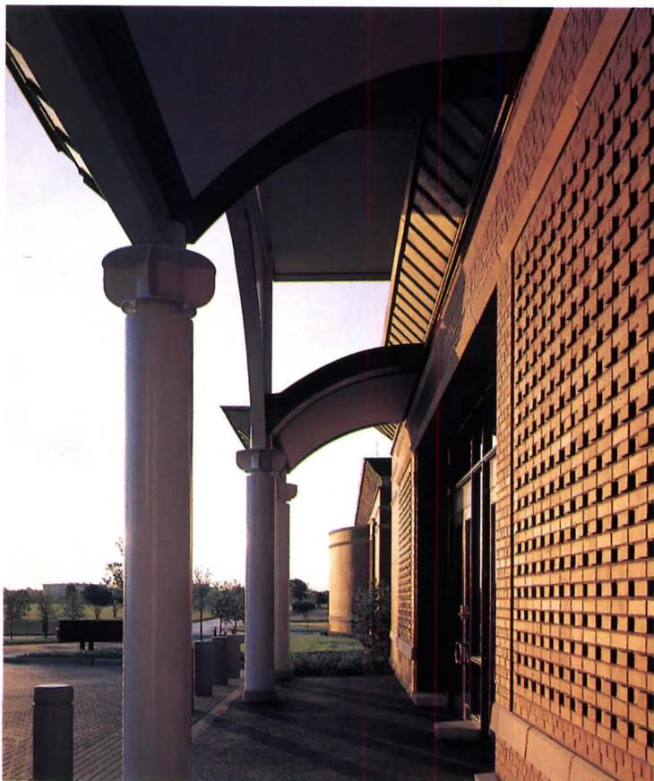
**Classically composed portico is sheltered by lead-coated-copper arched roof (below). Brick walls surrounding entrance (left) are variegated to simulate micro-chips by projecting every other brick in header course.**
