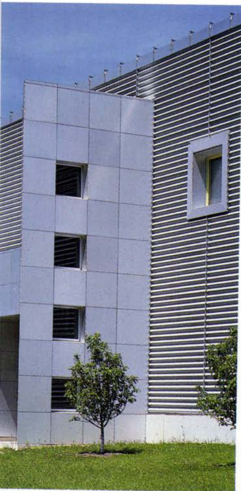
DETAIL OF CORNER AND SIDING DIVIDER
