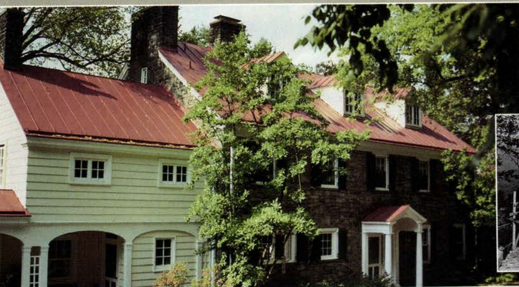
A standing seam roof of Follansbee Terne with over 62 years of service... still performing its designed function.
