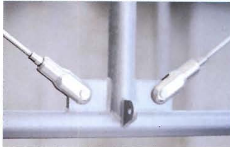
DETAIL: Stainless steel fittings connect rods and tubes.
