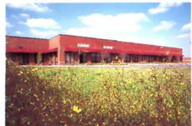
Independence Point Office Park, Charlotte, North Carolina, 17,000 sq. ft.; Architect/Engineer: Overcash/Demmitt; General Contractor: D. A. Davis Construction Co.; Steel Fabricator: Steelfab, Inc.; Steel Erector: Dixon Industries
