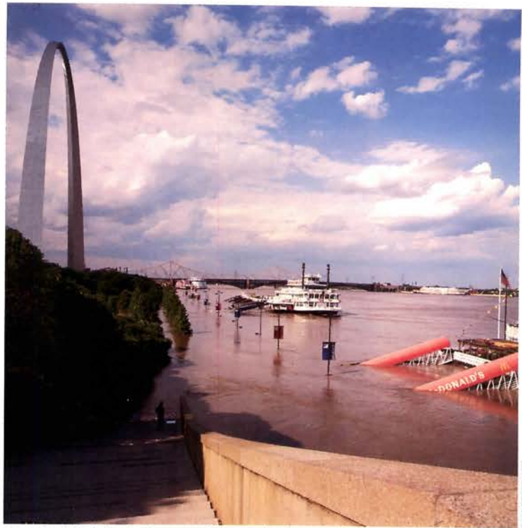
ST. LOUIS: Mississippi submerges Gateway Arch grounds and much of Eads Bridge.
