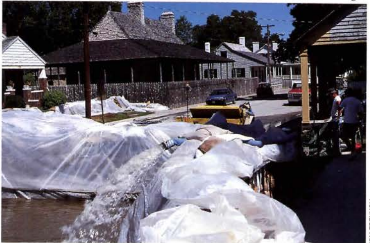
STE. GENEVIEVE: Sandbags helped to save 1770 Bolduc House and its fence.
