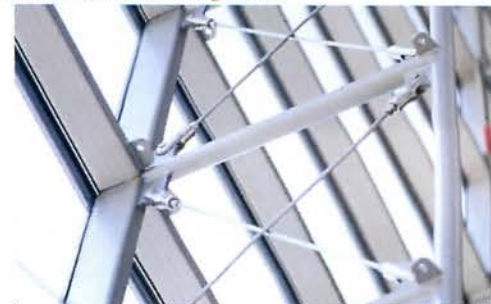
VERTICAL TRUSS: Tensile steel X-bracing.
