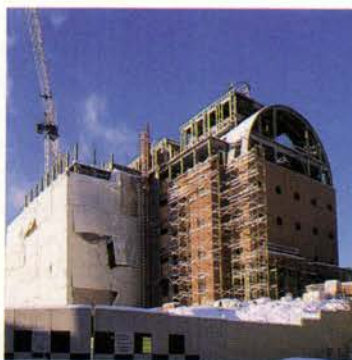
NORTHEAST CORNER: Steel truss vault.
