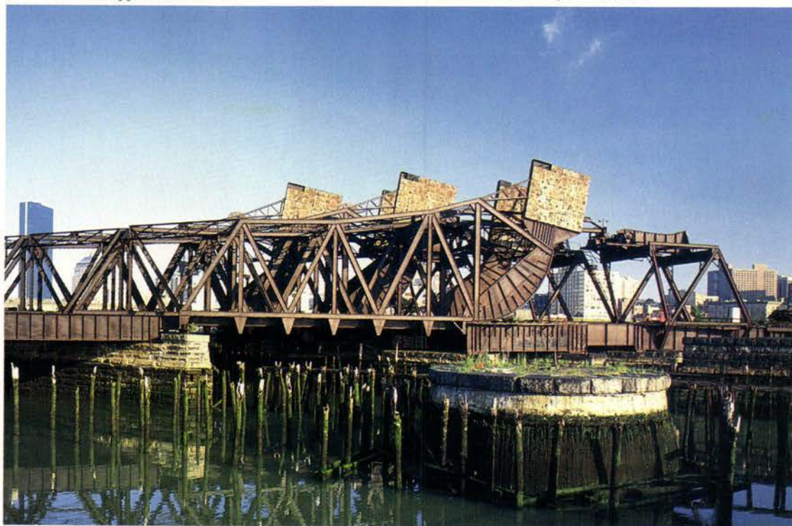
OLD COLONY BRIDGE: Counterweights and rocker arms (right) raise bridge span (left) over channel.
