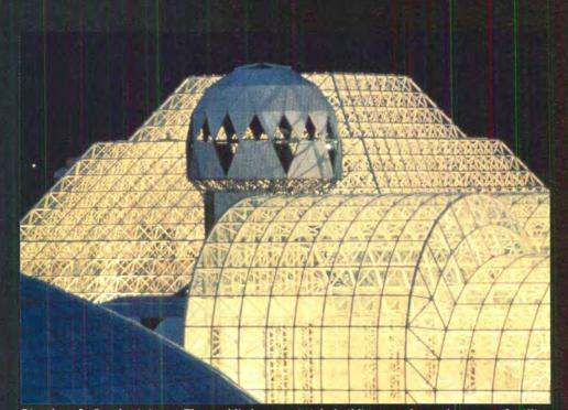
Biosphere 2, Oracle, Arizona. The world's largest airtight building complex encloses over 5 million cubic feet of volume. Both the structure and the glazing system were designed and manufactured by Pearce.
