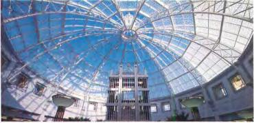
ROTUNDA: Fritted skylight reduces solar gain and increases thermal comfort.
