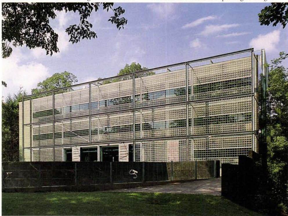
FINNISH EMBASSY: Heikkinen/Komonen's facade is screened by glass block and steel scaffolding.
