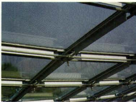
GLASS PANELS: Steel mesh filters sunlight.
