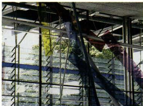
SOUTH FACADE: Glass louvers provide shade.
