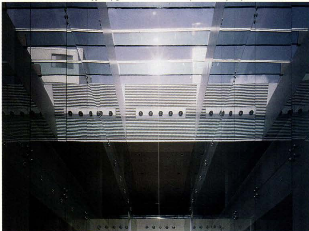
GLASS ROOF: Transparent roof introduces daylight into underground offices and offers views of Louvre.
