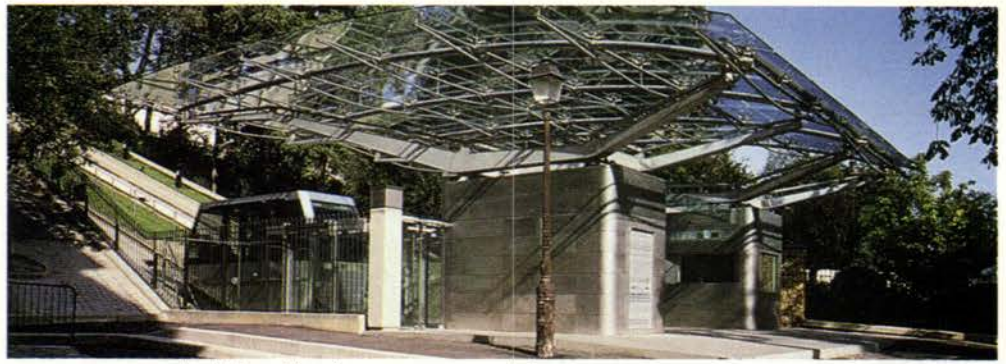
FUNICULAR STATION: Angled steel brackets support curved glass canopy.
