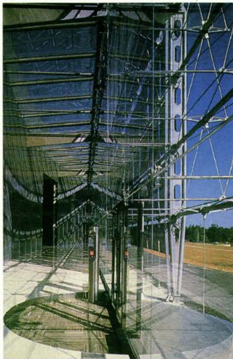
STEEL TRUSSES: Arms span between truss and wall.
