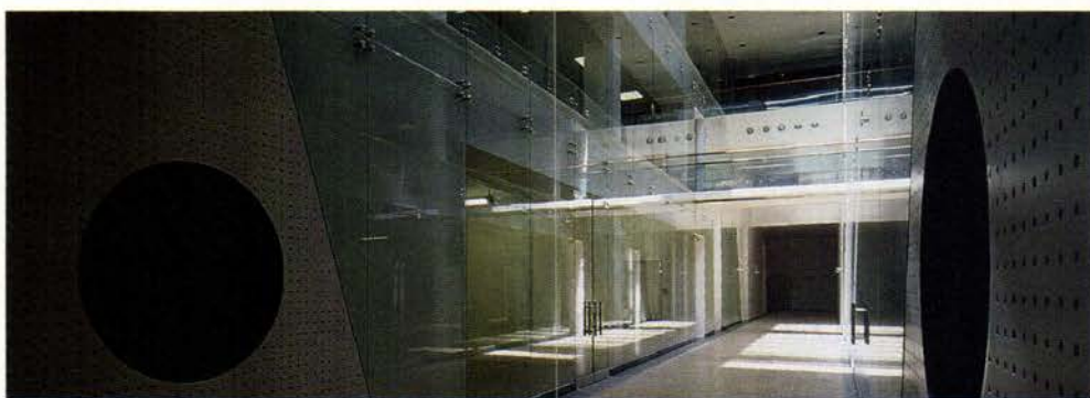
UNDERGROUND LABS: Atrium is topped by glazed roof and enclosed by laminated-glass partitions.
