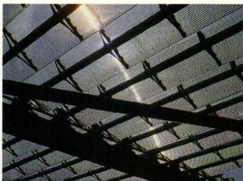
SKYLIGHT: Louvers regulate direct sunlight.
