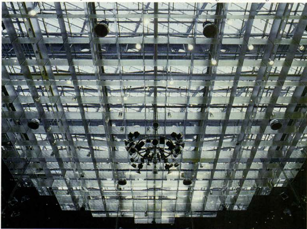
SKYLIGHT: Aluminum-and-glass baffles diffuse natural daylight in chambers of German parliament.
