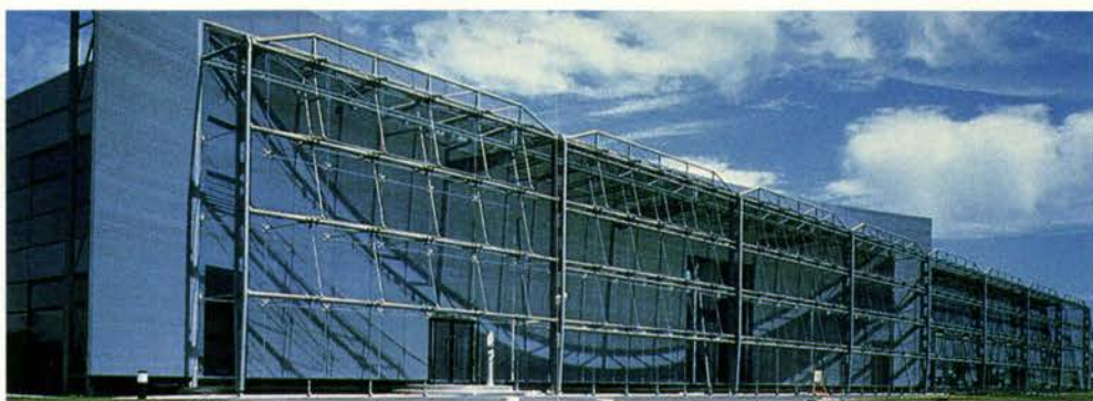
SOUTH FACADE: Steel trusses brace mullionless, laminated-glass panels.
