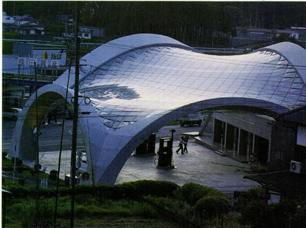
GAS STATION: Precast concrete arches support undulating glass canopy.
