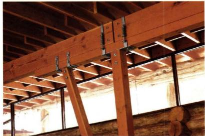
SPRING-LOADED SHRINKAGE-CONTROL CLAMPS AT DOUGLAS FIR COLUMN
