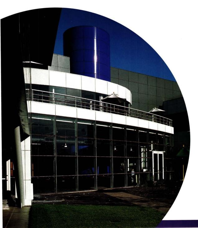
Dramatically marking the new Silicon Graphics Computer Systems demonstration center, San Francisco's STUDIOS Architecture chose ALPOLIC® aluminum composite material to clad over 36,000 ft<sup>2</sup> of wall surface and a bold 55-foot signature column.
