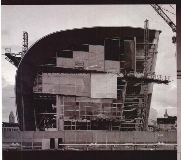
**Construction and** documentation difficulties were noteworthy because of the complex geometry of the building's double-curved surfaces. Initially, Holl wanted the great shell to be like the sides of a ship, sheathed in aluminum plates.
