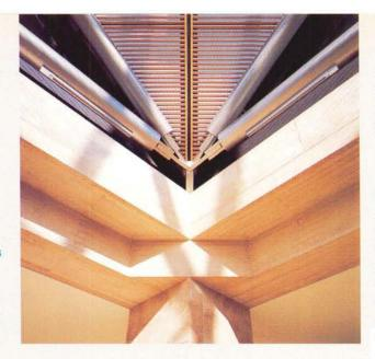
Space frame attaches to concrete wall through limestone cladding (right and below), face of which is on center line of space frame node.
