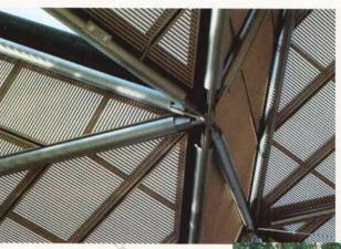
Typical space frame node (above and left) offsets glass and aluminum sunshade layers from structural chords. Peak of space frame (below) rises 14 meters above double-height tea court in south wing.
