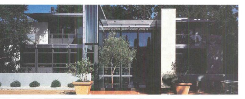
A custom glass curtain wall shaded by a steel brise-soleil encloses the house's rear facade (above). The glazed volume enclosing the circulation spine (see sidebar, facing page) projects beyond the patio facade, revealing the structure of load-bearing class channels. The architect feaves all joints between manmade materials exposed, as with the steel frame and C-shaped channel glass s
