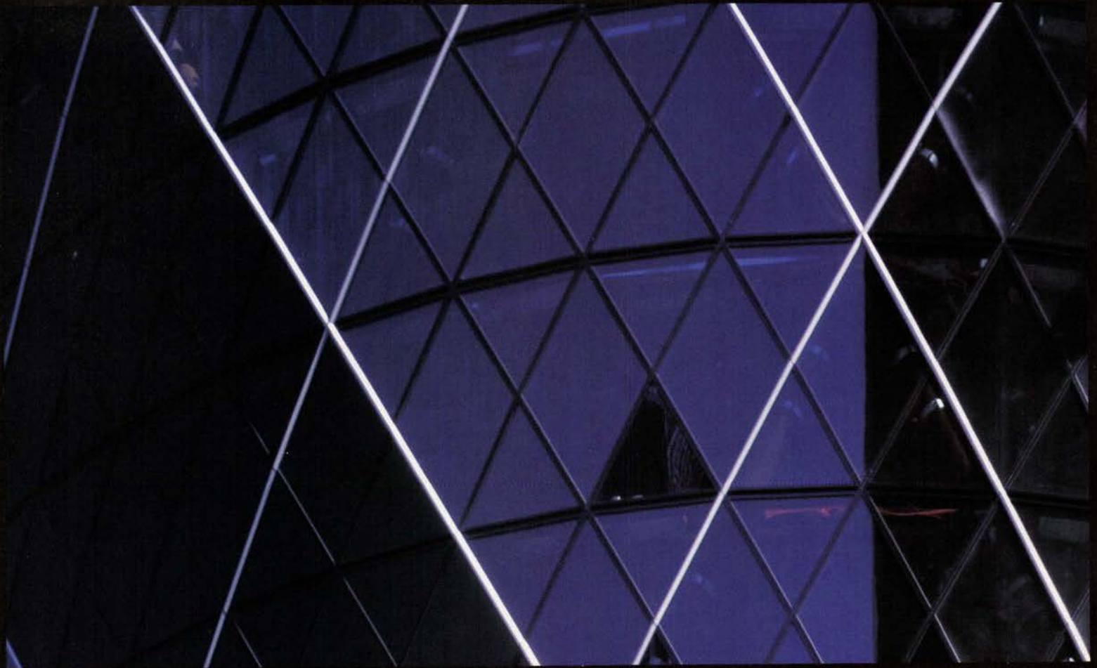
The 40-story Swiss Re, under construction in London, exemplifies the integration of structural and formal expression, long a hallmark of the work of its architect, Foster and Partners.
