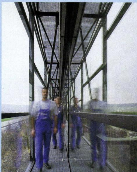
**A double façade (above) combines emergency egress with a passive climate control system of louvers and vents. Precast concrete panels cover the base and side walls (facing page).**
