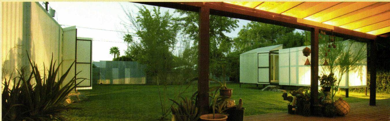
SUPPORTED BY BOULDERS BURIED IN THE GROUND, THE BACKYARD SLEEPING PODS ARE ALSO MEANT TO BE MOBILE—THEY CAN BE REUSED AS SHIPPING CONTAINERS FOR THE OWNER'S BELONGINGS WHEN IT COMES TIME TO SELL THE HOUSE. AIR CONDITIONING AND ELECTRICITY IN THE PODS ARRIVE THROUGH A STANDARD EXTERIOR OUTLET.
